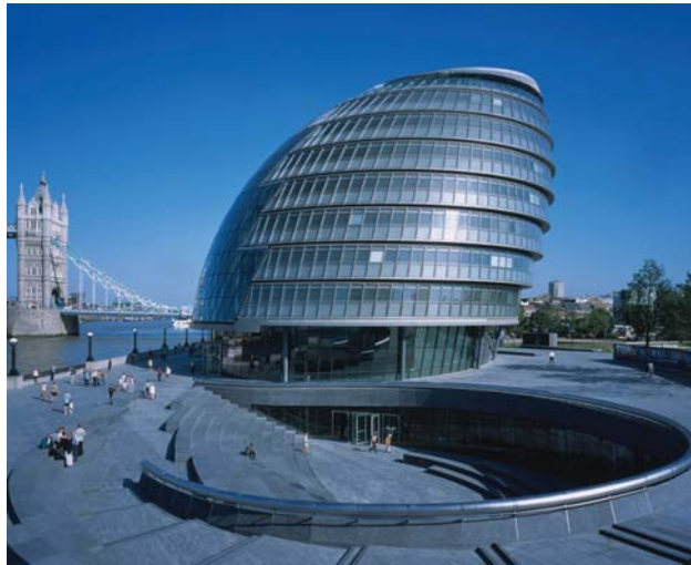
15.14 The City Hall in London (1998– 2002), architect Foster and Partners, engineer Arup.
