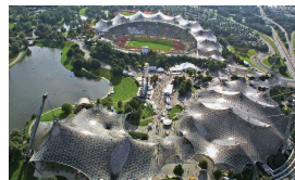
Munich Olympic Stadium (1972)
