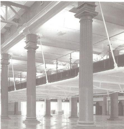
The Billingsgate Market Refurbishment, London, Image from Connections: Studies In Building Assembly ,
